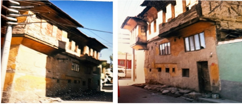
Figure 5. Rear façade prior to restoration (Eskişehir Council for the Protection of Cultural and Natural Assets, n.d.).
