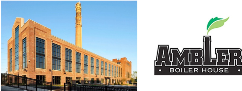
Figure 9. The Ambler Boiler House building and logo (Ambler Main Street, n.d.).
